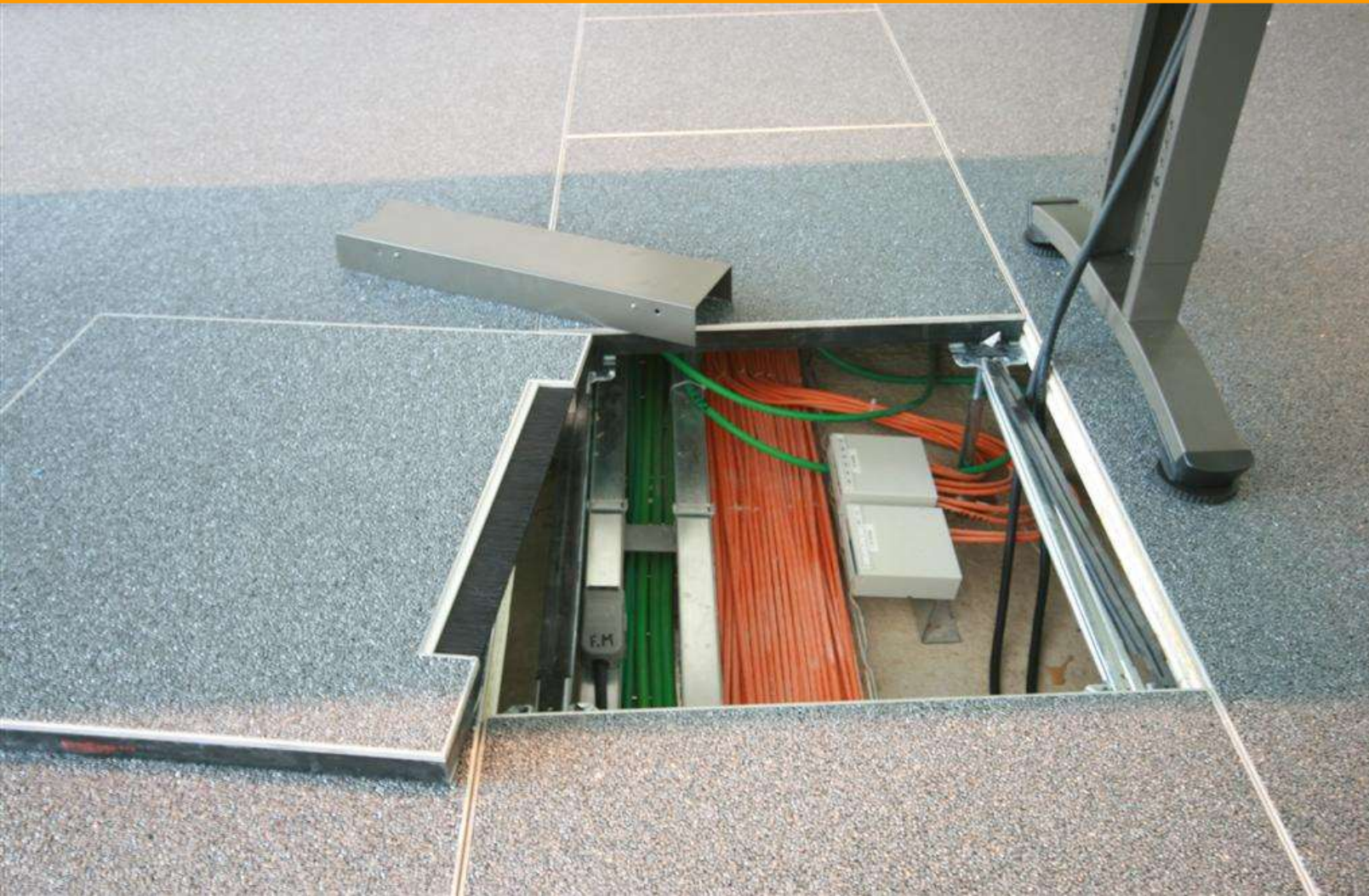
accessible panel for local electrical outlet
