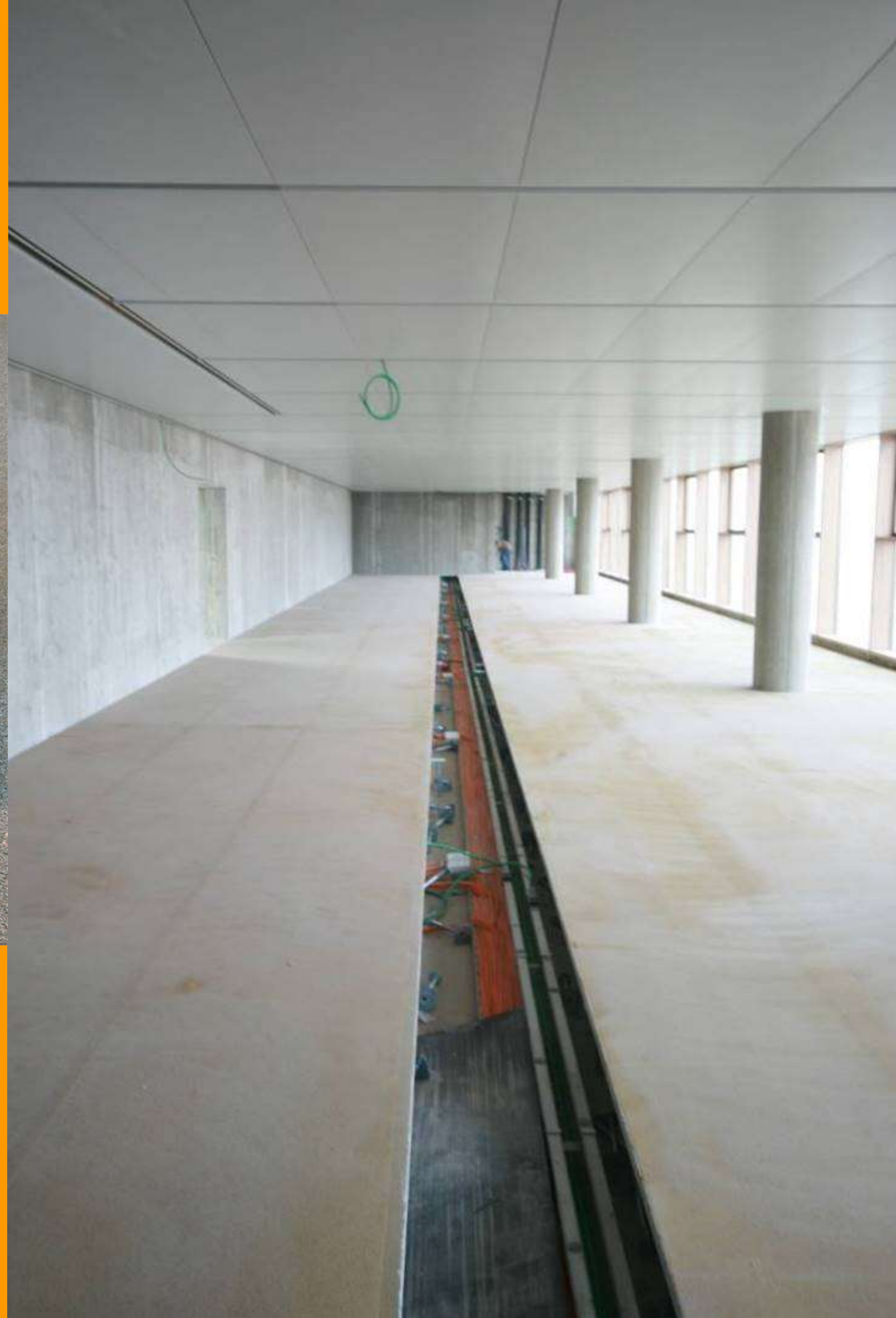
accessible panel for local electrical outlet
